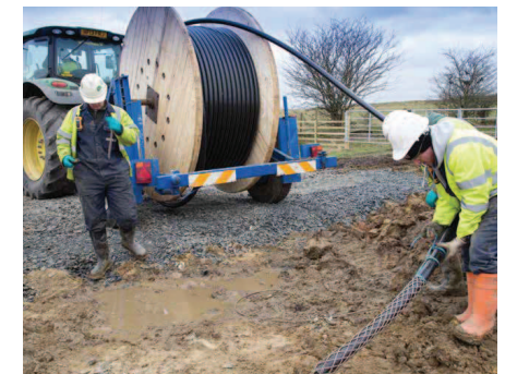
7. Pull cables into ducts
